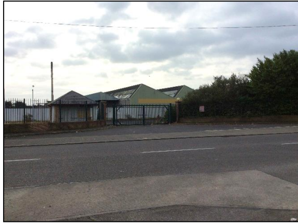
Figure 2.3 Existing Access off Coolock Drive
