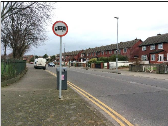
Figure 2.4 Greencastle Road Facing East showing junction with Coolock Drive
