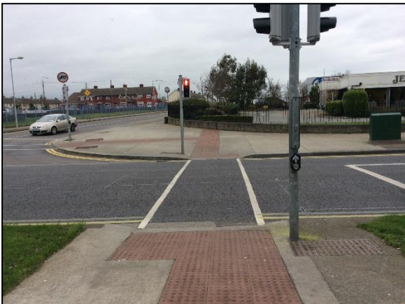
Figure 2.6 Existing Pedestrian Crossing on Oscar Traynor Road
